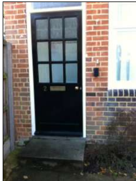
Front door with key safe to right
